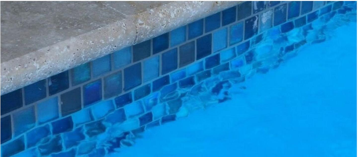
Waterline or perimeter tile is ceramic or glass tile fixed to the surface of a fiberglass pool with waterproof silicone adhesive. The adhesive and its accompanying silicon-based waterproof grout will allow waterline tile to flex and move with the pool shell.
