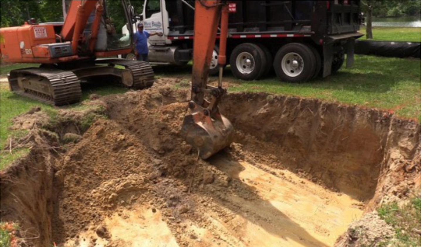
The first thing we'll do is **"paint" the pool on the ground** and **use a laser level** to establish how high to set the pool in the yard. **This tells us how deep to dig.** A dump truck will be moved close to the hole if needed before excavation begins.
