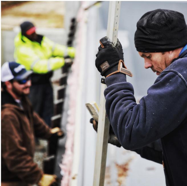
**The entire pool floor must rest on a solid foundation to keep it structurally sound and prevent shifting and settling over time.** Our crews aim to get your pool to within half an inch (or less) of level or less, while ensuring its entire floor is firmly on its foundation.
