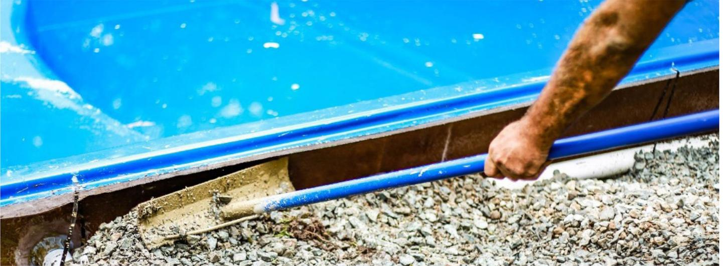
Once plumbing is done, and the pool shell is set and leveled, it's time to **fill the pool with water** and **backfill the perimeter with gravel**.
