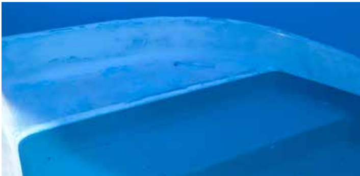
Examples of discoloration in fiberglass pools
