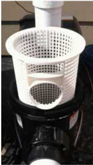
Strainer pot basket (located in the end of the pump)
